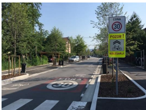
Figure 6: Cesta zmage after renewal (photo: Kaja Pogačar)
