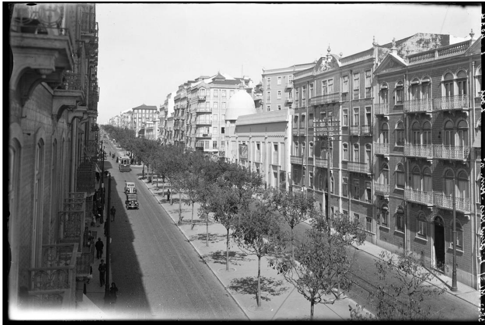
Figure 4: Initial type section partition of the Avenue, already with the introduction of trams (Eduardo Portugal, 1938). Arquivo Fotográfico Municipal: PT/AMLSB/POR/021056
